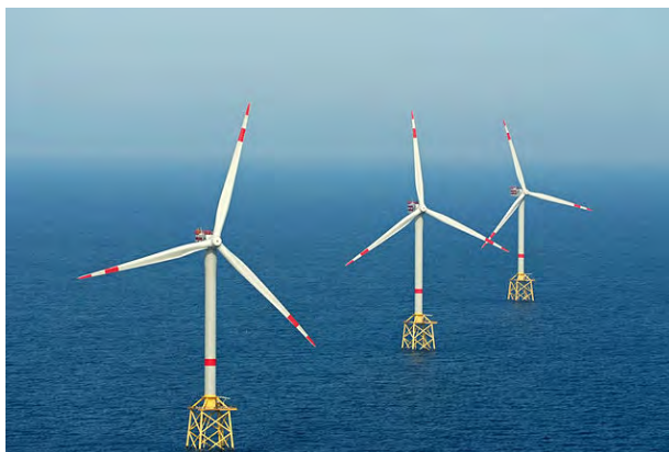
Figure 2.4 Examples of Turbines on a Jacket Structure
