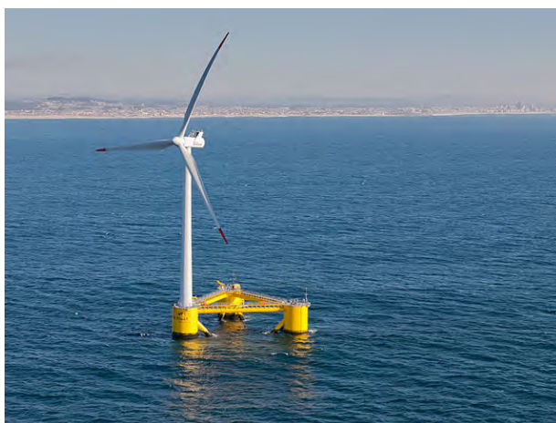
Figure 2.5 Example of Floating Wind Turbine - Windfloat by Principle Power
