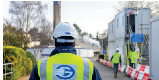
Site visit of the new Substation works at the Princess Elizabeth Hospital
